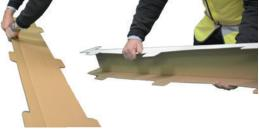
3. Pre-bend the two cable tray components along the scored lines.
